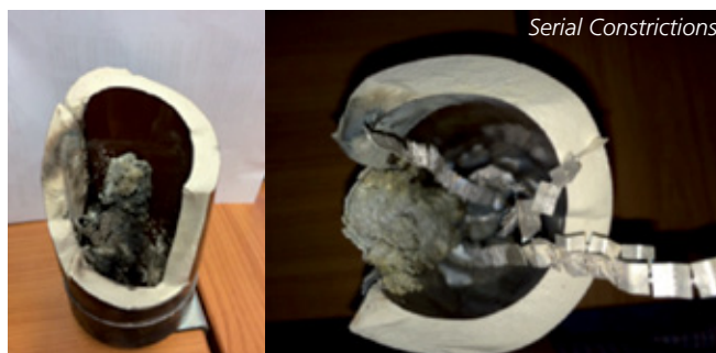
View of a failed / ruptured fuse
