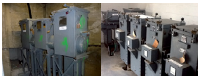
View of Long & Crawford ETV3 oil filled switch arrangement (A high percentage of these have been used in underground substations as shown above)
